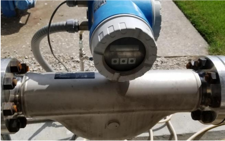
Figure A.3 Coriolis Flow Meter
